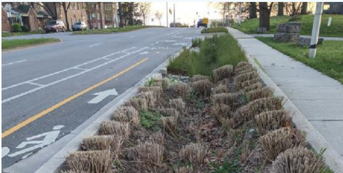
A bioretention facility on Liberty Heights Avenue.
